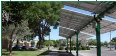
The structure will provide shade for cars and track the sun to ensure maximum light and maximum output of electricity.
